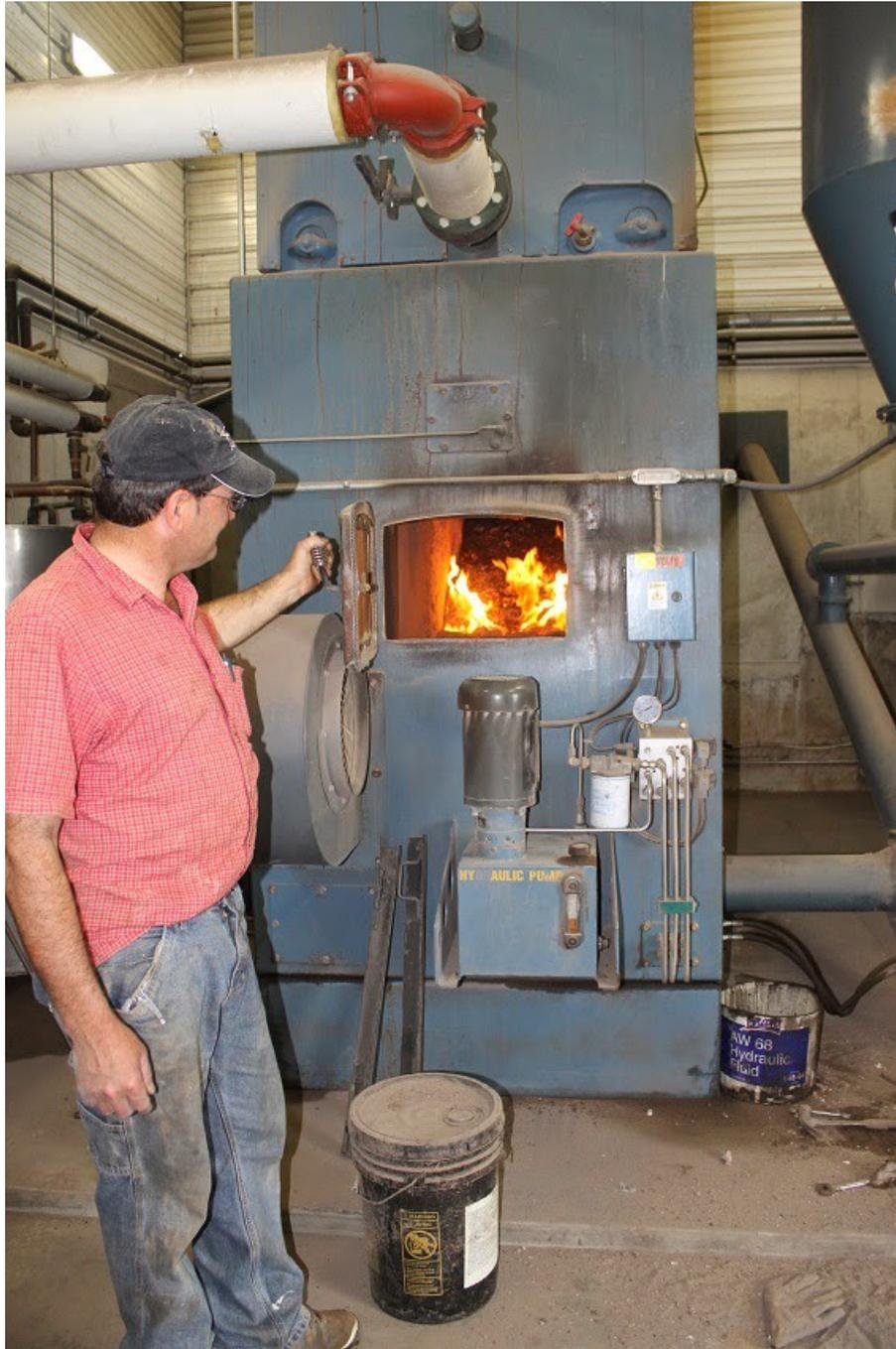
Earl Ray showing his new and unique furnace for burning chicken manure to create hot water to heat the chicken barns. See [www.BlueFlameStoker.ca](http://www.BlueFlameStoker.ca) for more information.
